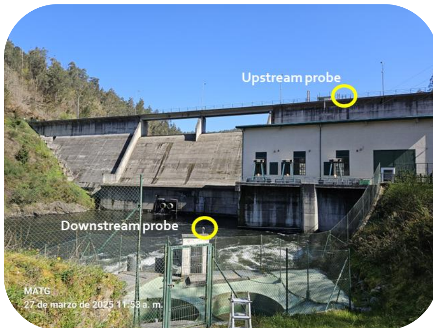
Figure 1: Salto de Touro Hybrid HPP, Spain
